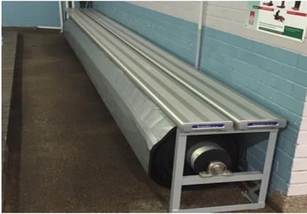
Have you noticed the new sparkly metal seating down on the pool deck? This is home to one of our new pool blankets. We have installed these blankets to help maintain continuity in water temperature. These blankets conceal the heat
